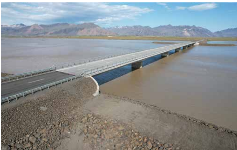
4 Bridge over Hornafjarðarfljót © IRCA
