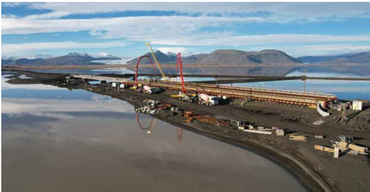
12 Concrete works for Stage 2 of the bridge over Hornafjarðarfjót © IRCA
