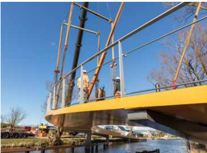
4 5 6 Lifting and assembly of the prefabricated steel structure © ipv Delft
