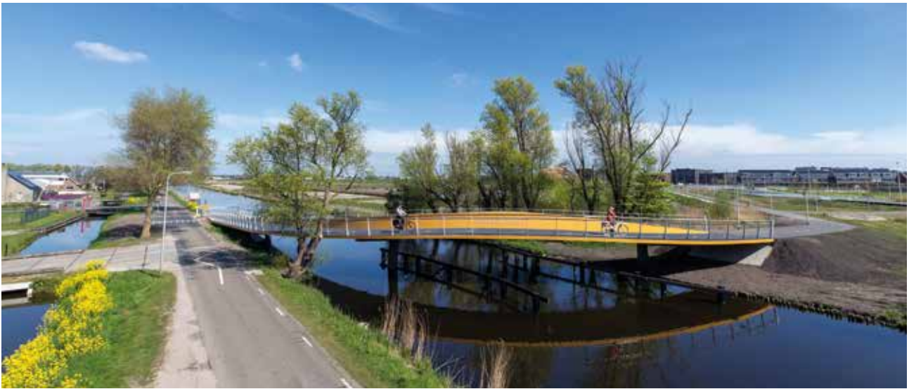
12 New canal crossing for cyclists upon completion © ipv Delft
