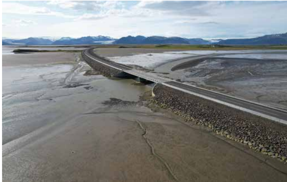
5 Bridge over Bergá © IRCA
