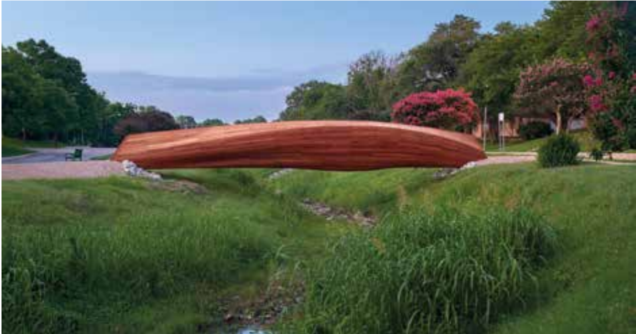
1 Ship hull shaped bridge over the small creek © Peter Molick
