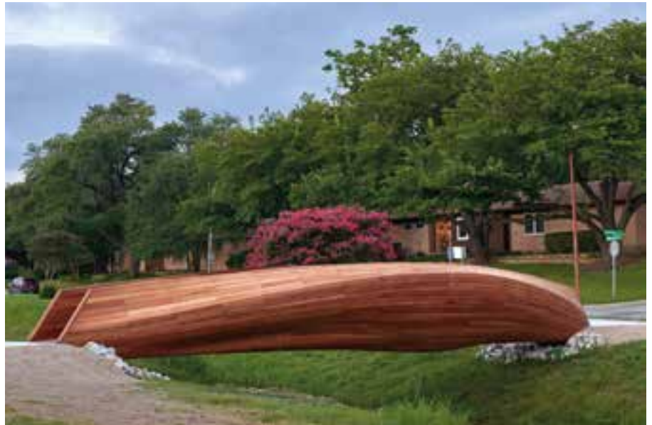
21 Connecting element between two neighborhoods © Peter Molick
