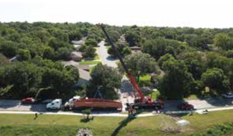
19 20 Lifting of the pre-assembled bridge onto the bearings © Raymond Cervantes
